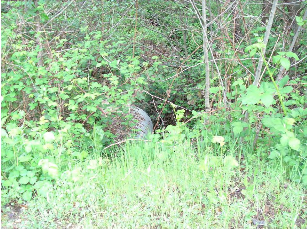
Photo 6: Culvert and drainage downstream (west) of dirt road (DR-5).
