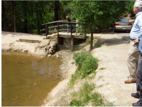
Figure 4. Lumsden Lake culvert.
