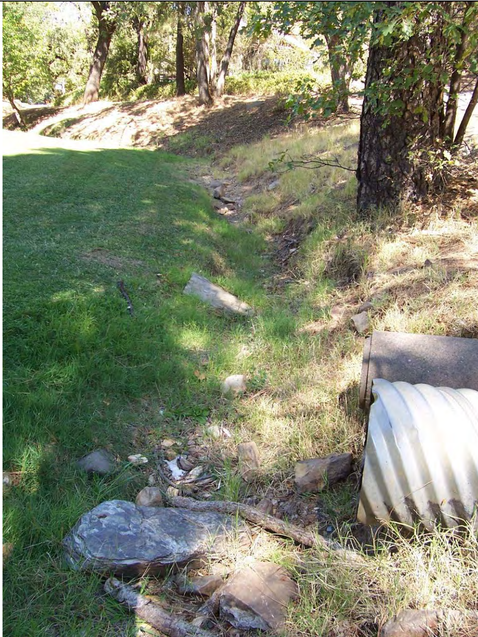
Photo 5: Modified channel downstream of 5-acre parcel, at Lumsden Park.
