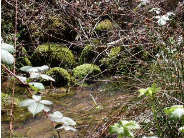
Figure 2. Open area of drainage with 4" of water
